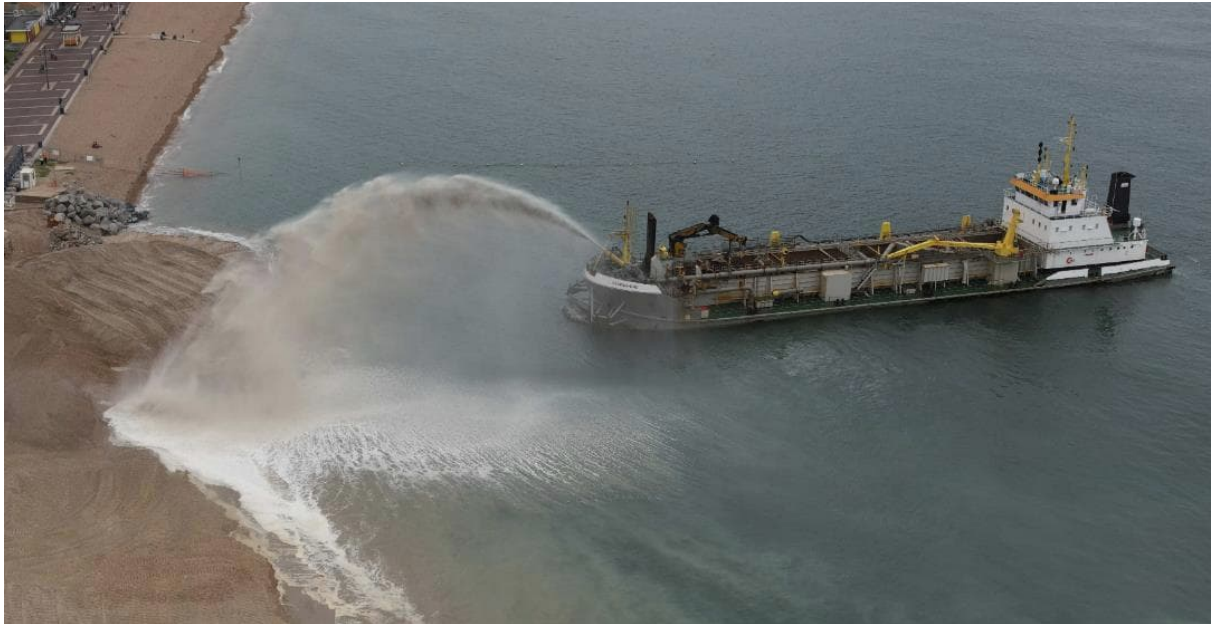
Figure 1 Sospan Dau "rainbowing" material ashore.
